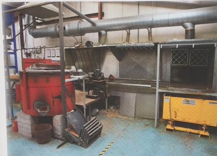
Here you can see the furnace (red) with the rollers behind on which the moulds are moved as they are filled.
